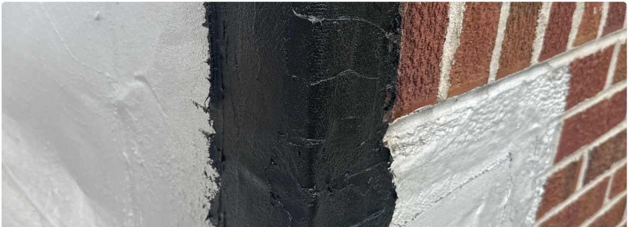
Repair performed — open wall flashing at brick corner sealed full height
