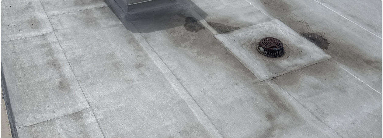
Elevator shaft roof — smooth membrane, newer and in better condition; one drain with rusted strainer
