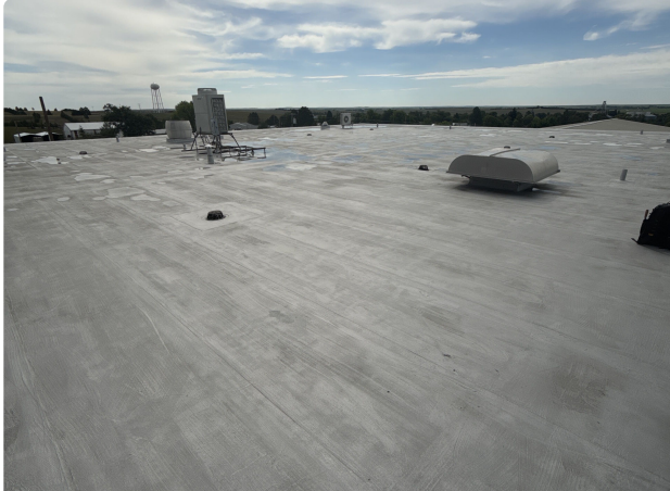
Elementary roof overview — modified bitumen with aluminum coating, HVAC curbs, drains and prior patching
