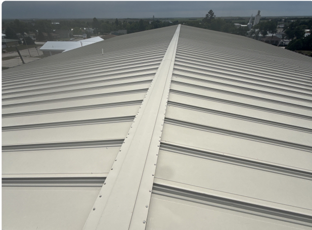
Community Building overview — metal roof, relatively new and in good condition
