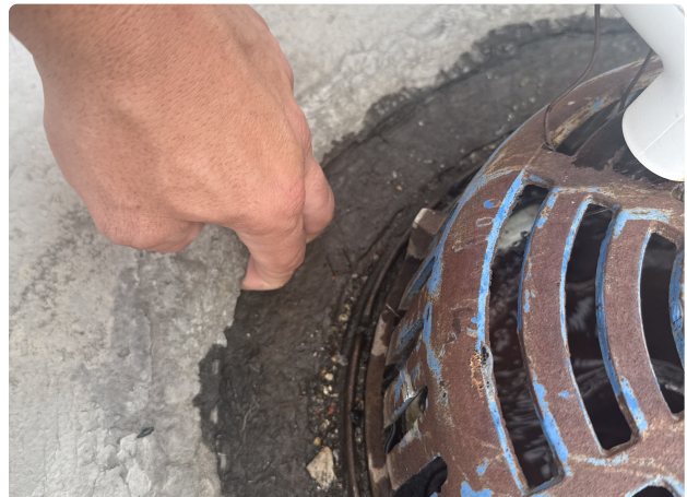
Second open target patch at drain sump
