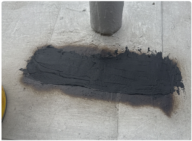
Repair performed — mastic repair at open base tie-in seam
