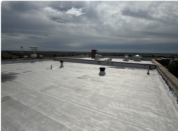
Third floor overview — more uniform condition than the Elementary and North sections
