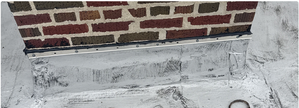
Repair performed — silicone removed, term bar cleaned and resealed with compatible sealant
